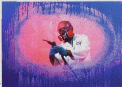
Photo 1—Spraying Grancrete on a panel
