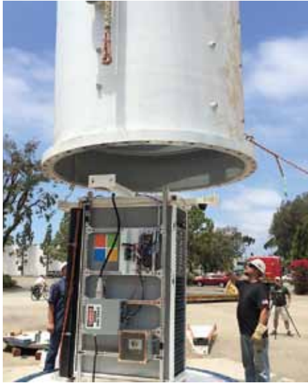
Photo 3—The team not only developed the vessel concept, they also had to determine how much hardware you can safely stuff into its limited space.
