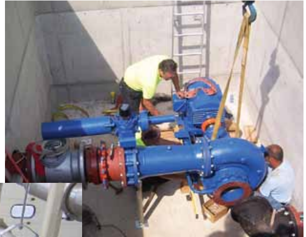
Photo 1— Westmoreland County pump station installation
