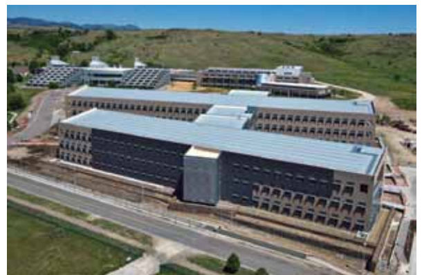
Photo 2—To maximize sunlight entering the building, each section of the facility is only 60' wide.
