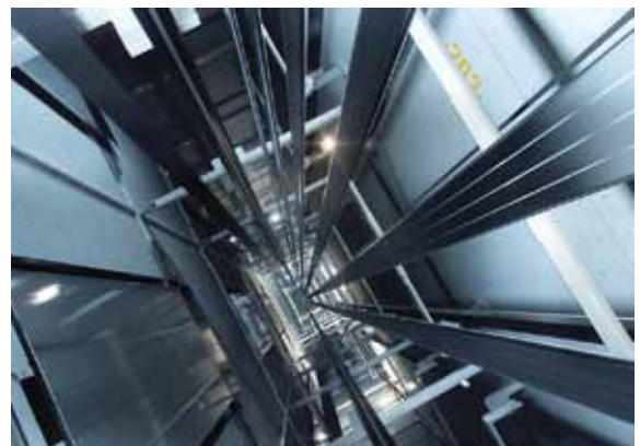
Photo 3 (above)—Elevators that travel in very tall skyscrapers slowly accelerate and slowly decelerate to keep their occupants comfortable and safe during the ride.
