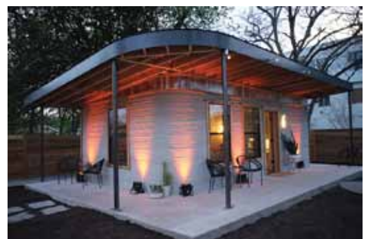
Photo 3 (above)—It only took 47 hours for a 3D house construction printer to build this house.
