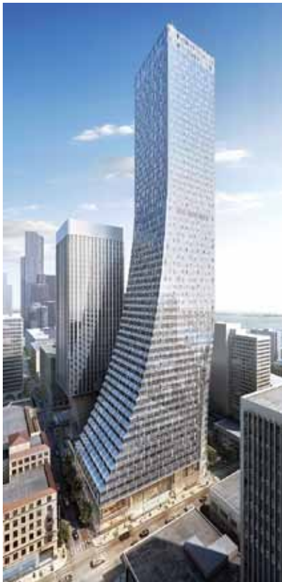
Photo 1—The Rainier Square Tower, under construction in Seattle. The construction is using the new SpeedCore building system to construct the building's core superstructure. This technology will cut construction time by about 40%.
