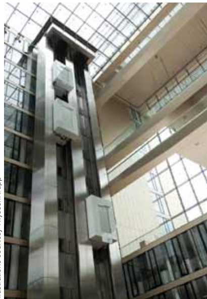
Fig. 1—The TWIN elevator system has two elevator cars running independently in the same elevator shaft.
