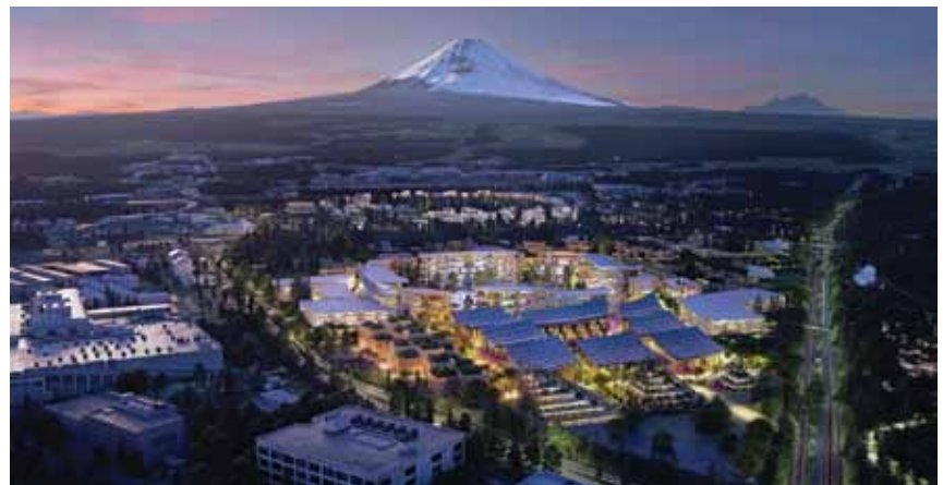
Photo 2—An architecturally rendered aerial image of the Woven City that will be built at the foot of Mt Fuji in Japan.
