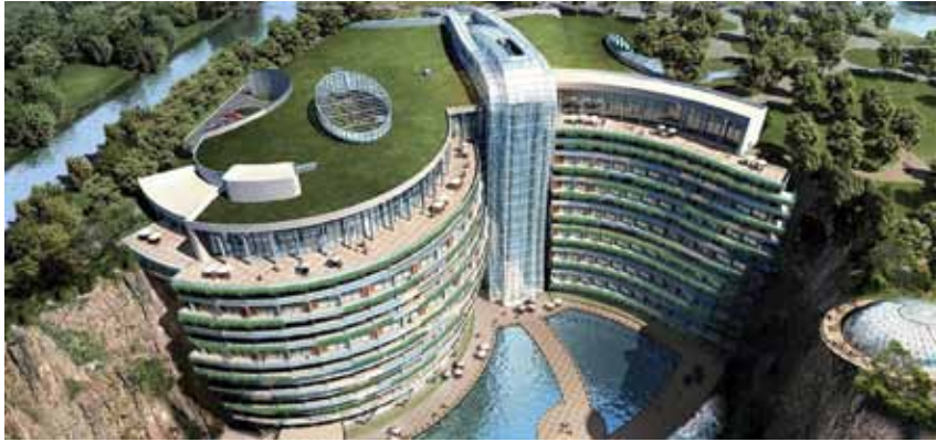
Photo 3—Architecturally, the Shimao Wonderland Hotel in Shanghai is in total harmony with its surroundings. It brings new purpose and value to an abandoned rock quarry.
